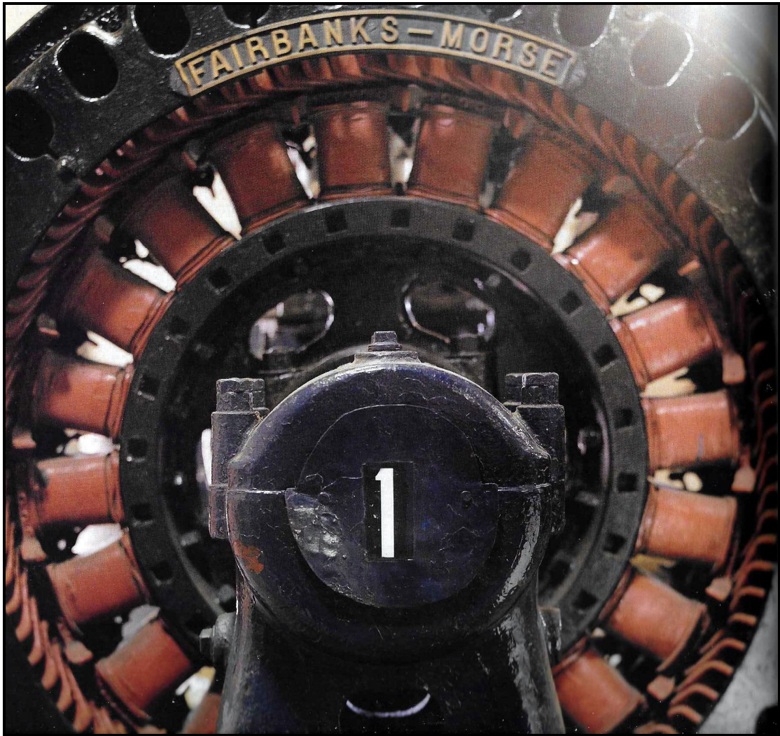
Fairbanks Morse armature of a 1940 Frick 10 x 10 ammonia compressor Pascagoula Ice & Freezer Company
